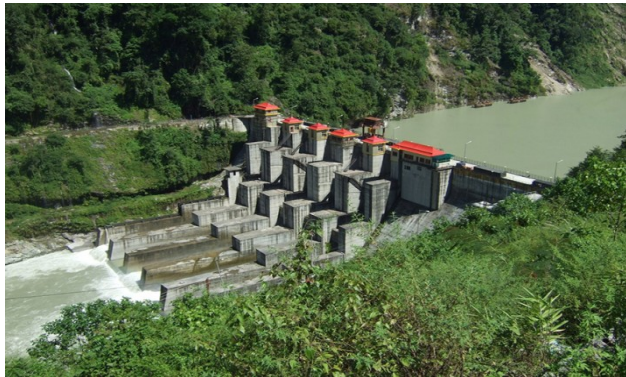
Teesta-V hydropower station, Sikkim Photo: Hydropower.org
